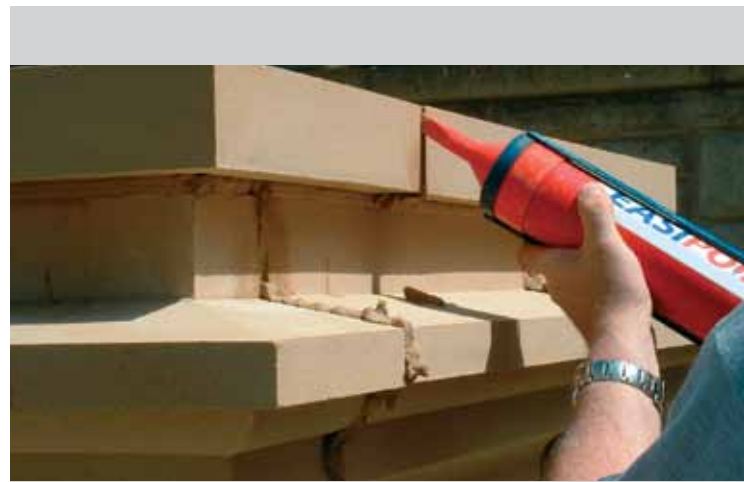
Easipoint mortar during installation.
